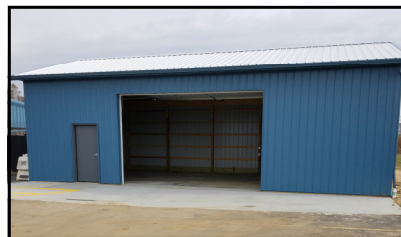
Brand new pole building
